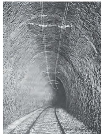
Figure 3: The historic three-phase over-head contact line in the Simplon tunnel.
